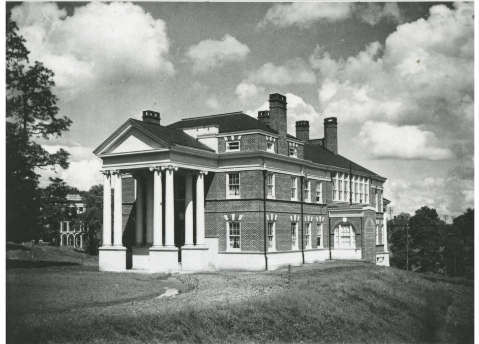
Administrative Wing of Hospital, 1901. Note the hyphen to link to future South Wing. Historical Collections & Services, Claude Moore Health Sciences Library, University of Virginia.
